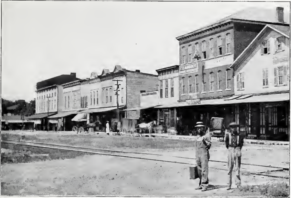
NORTH RAILROAD STREET. OSBORN. Under the plans of the Conservation District, this town will be removed.
